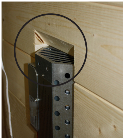
Fig. 1: Do not cover ventilation slots
